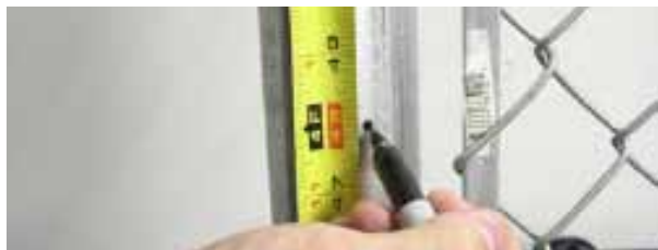
Measure up approximately 4ft for the first mark
