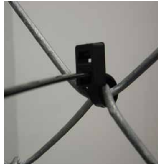
STEP 1 SHOWN BEFORE SENSING FIBER IS INSTALLED
