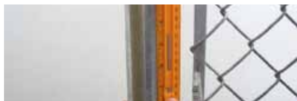
Measure 7 1/8" above the first mark and make second mark
